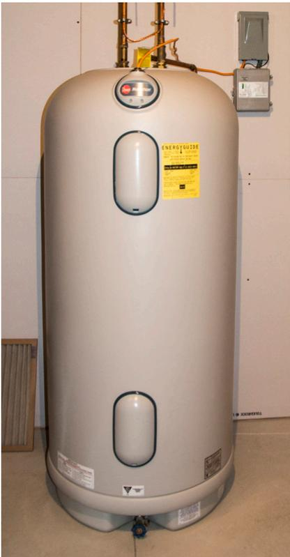
The LCT is pictured here in the upper right corner. In this set-up, the member’s water heater is connected to the LCT.
