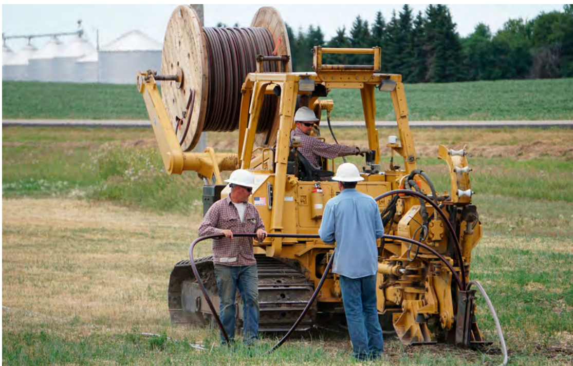
Verendrye linemen install new underground power line in this photo. Verendrye has about 4,619 miles of power lines with about half of it buried under ground.
