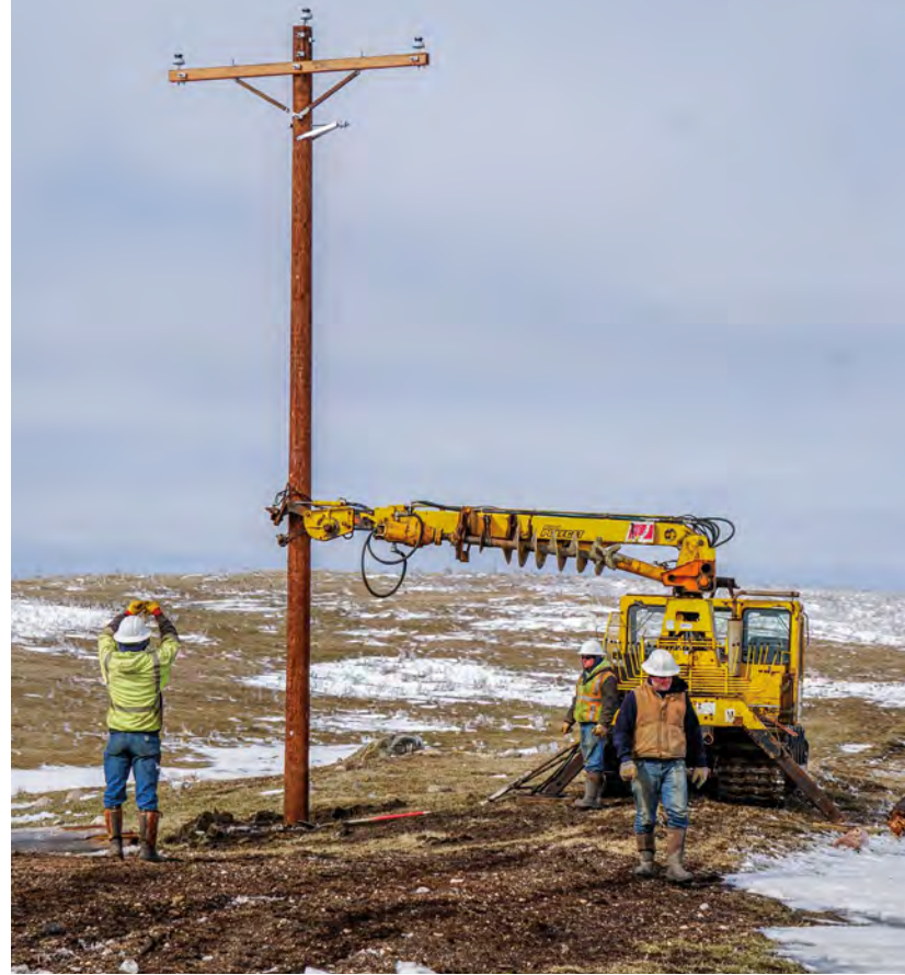
Lineworkers install a new pole after the April 2022 ice storm that broke 478 poles, causing 2,000 members to lose power.
