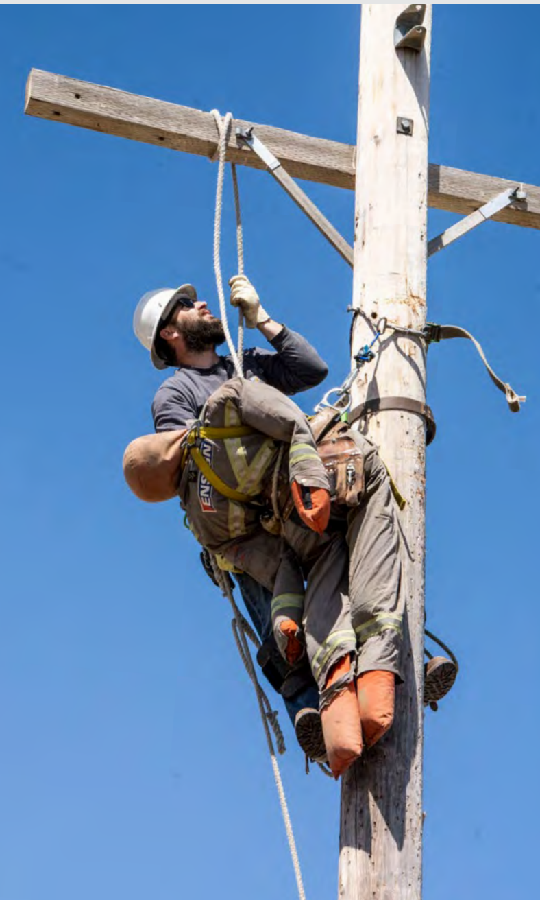
Lineworker Nick Pfau performs a poletop rescue training exercise. All lineworkers are trained to be able to climb a pole and rescue another worker if necessary.
