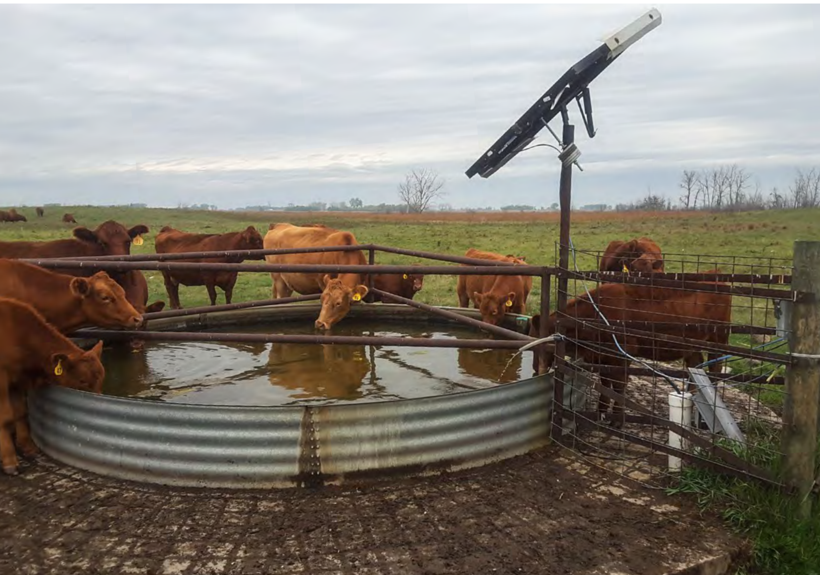
Cattle drink water that was pumped from a well using one of Verendrye's 300 solar systems that ranchers can rent.
