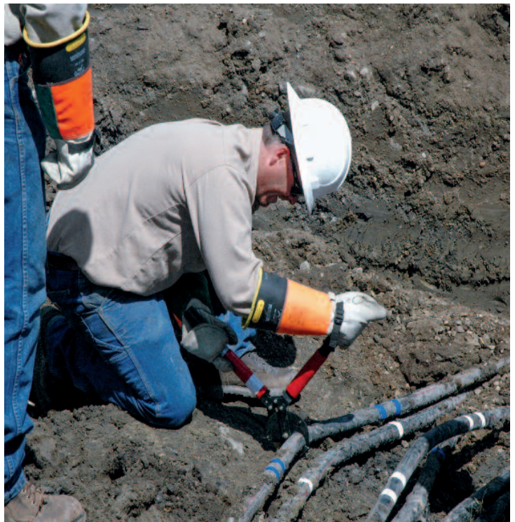
Verendrye lineworkers repair an underground power line after it was damaged by a backhoe. Hitting an underground power line can be dangerous and can also cause outages.
